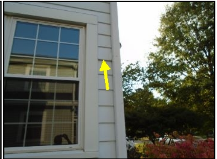
Location of previous photo.
