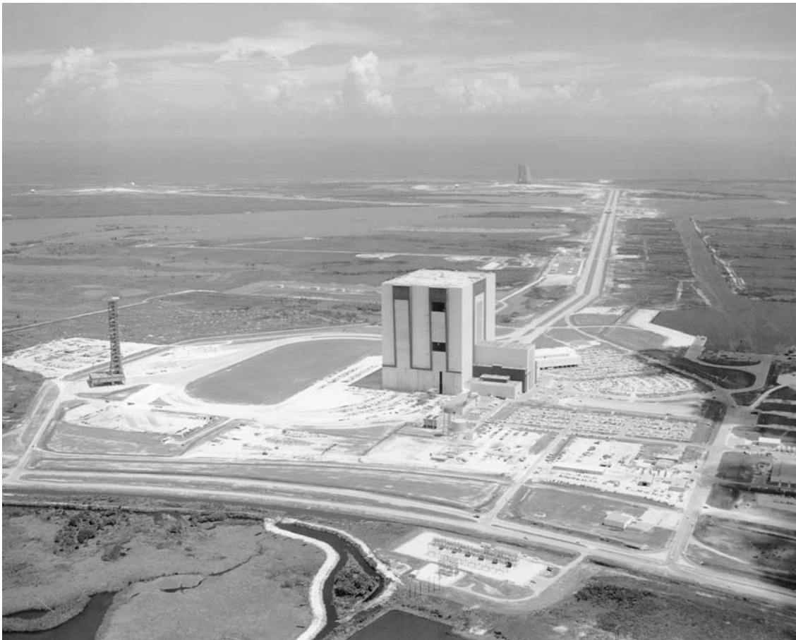
FIGURE 4. Heavy construction project—Kennedy Space Center launch complex. (U.S. Air Force photograph)
