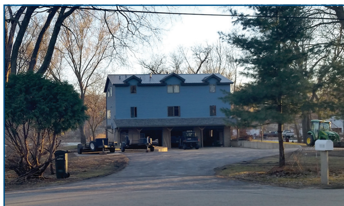
Figure 1: This home along the banks of the Cedar River has been raised so that flood waters no longer reach the main floor during flooding events. The lower area is used as a parking area and has flood damage resistant construction materials (Cedar Falls, Iowa)
